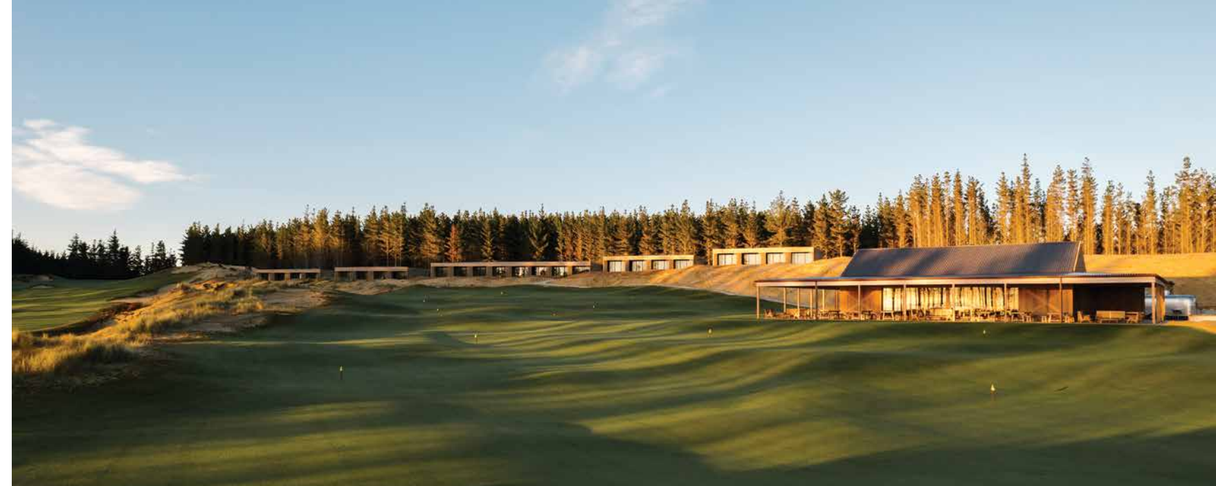
Te Arai’s suites and two-bedroom cottages have interiors by noted US designer Jenni Kayne.
